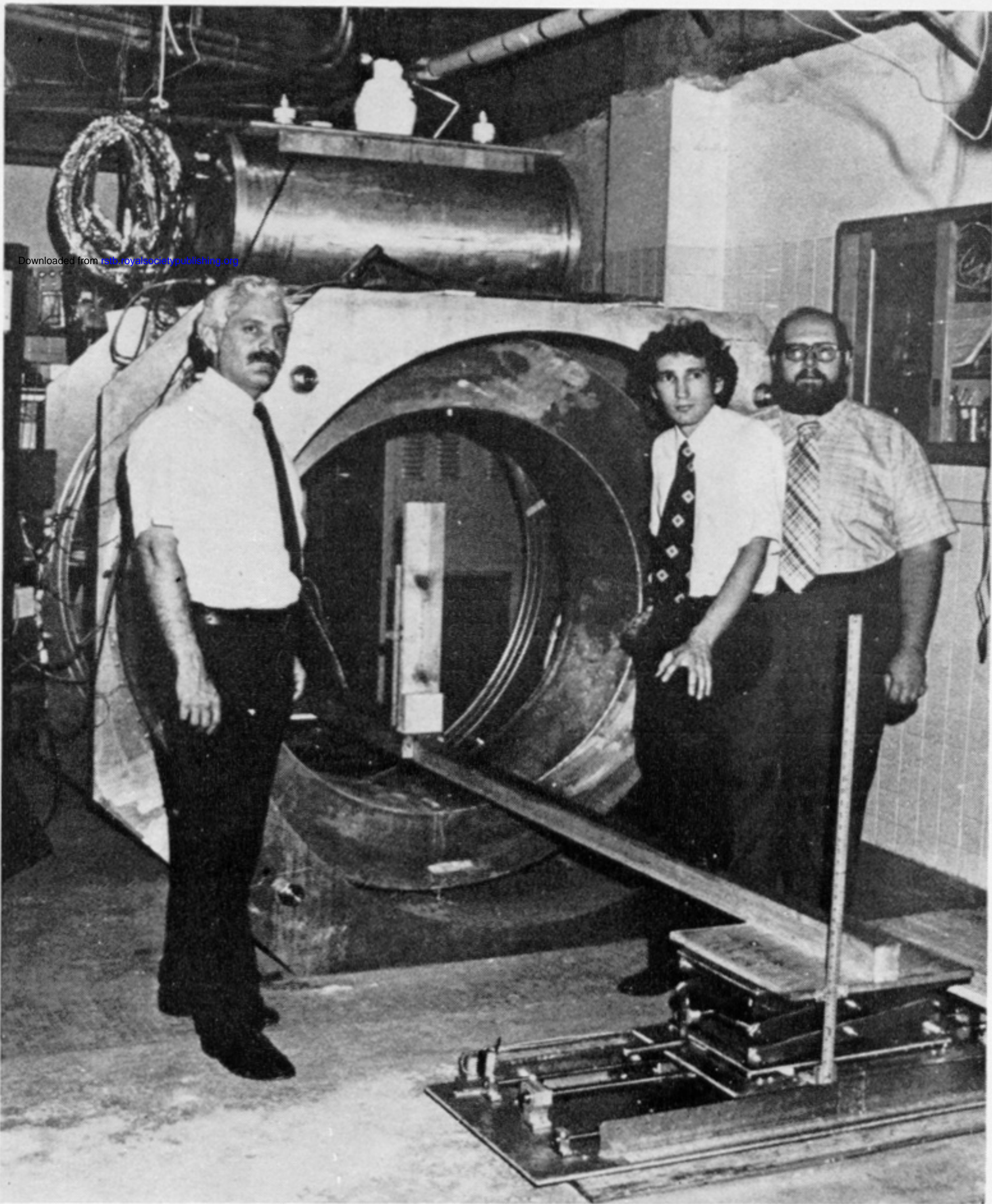
FIGURE 7. Completed human n.m.r. scanner. (Left to right) Dr R. Damadian, Dr. L. Minkoff and Dr M. Goldsmith.
